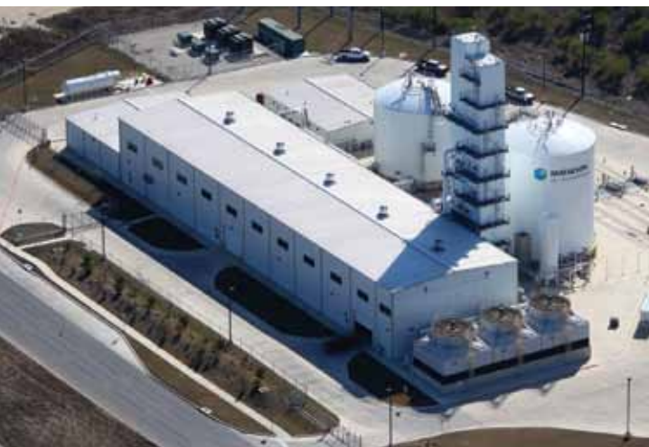
MATHESON Air Separation Unit, San Antonio, TX
