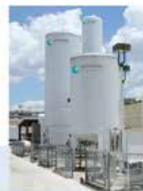
Onsite & Pipeline Plants
