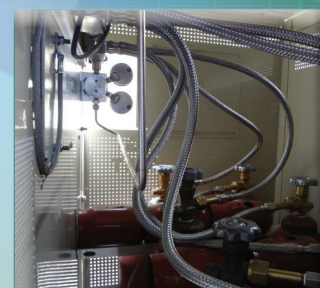
Fuel Cell Hydrogen Source Manifold
