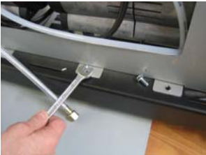
Fig. 8-6 – unscrew bolts from compressors
