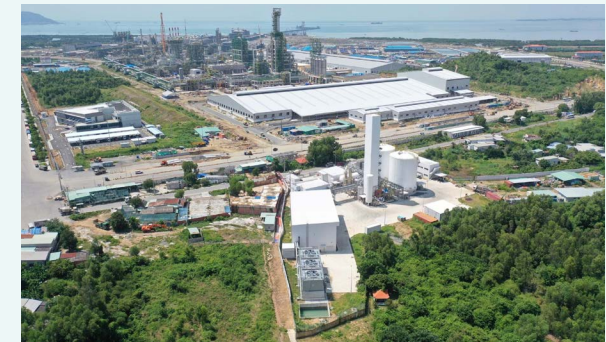
Plant using remote IO technology
